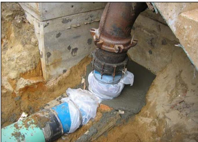
The 16" rapid sand filter backwash drain line is now connected to the PTR facility where all backwash water is captured and recycled. This is not only better for the environment, but allows the District to utilize its more efficient rapid sand filters on a continuous basis. Recycling operations began on April 24th, only seven weeks after the start of construction.
