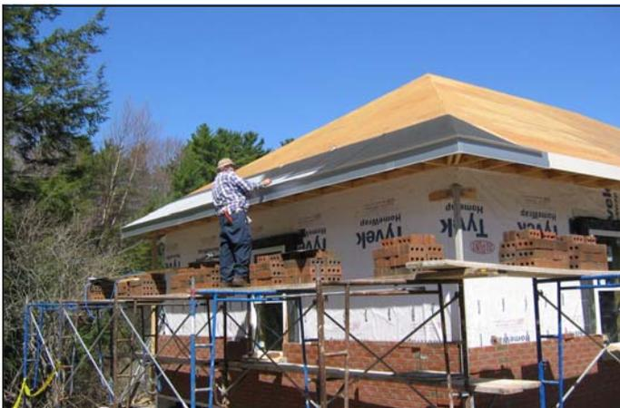
The PTR facility's roof shingles and brick facing are designed to complement the District's adjacent treatment plant buildings along Rte. 1 at the Kennebunk-Wells line. A private contractor was hired to construct the building shell while District crews are responsible for all plumbing, electrical, HVAC, controls, finish work in addition to installing all exterior piping and site work.
