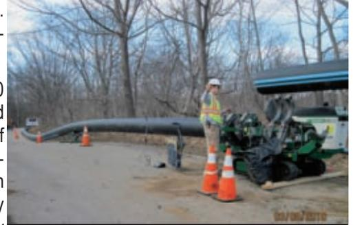
16" HDPE pipe is fused and strung out in advance of a directional drilling (DD) operation on Skipper Joe's/Marshall Point Road in Kennebunkport. DD is a form of trenchless technology that minimizes soil disturbance when working around environmentally sensitive areas such as salt marshes and wetlands.
