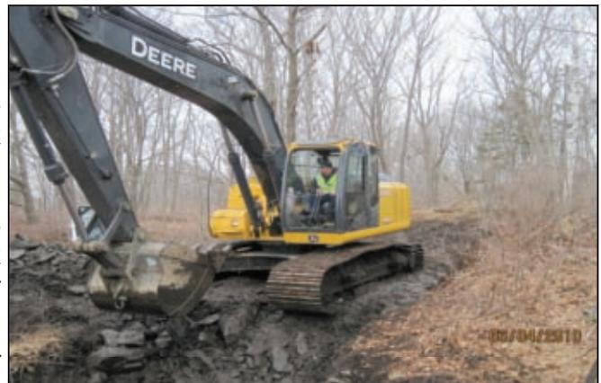
The District's Shane Batchelder begins excavating a trench in early March for the new 16" ductile iron (DI) water main on Skipper Joe's Point Road in Kennebunkport. This \$2M federally funded project is expected to take six months to complete and includes replacing over 10,000 feet of obsolete 10" cast iron pipe with new 16" DI pipe.
