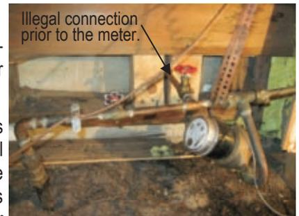
The District recently discovered this illegal plumbing configuration where an illegal connection was plumbed prior to the meter. By connecting a hose to this illegal connection, the customer was using unmetered water for irrigation. The District views water theft as a serious matter that can result in the water service being disconnected along with the customer being assessed a hefty fine. Promptly report any suspected water theft to the District to better protect all customers.
