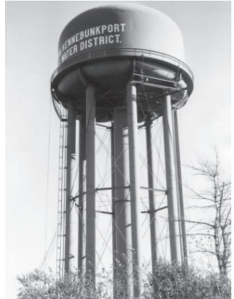
Photo of the Cape Porpoise (a/k/a Crow Hill) water storage tank after construction was completed in 1954. Despite the harsh salt water environment, the useful service life for this steel tank should be well over 100 years with proper care and maintenance. So this local landmark should be around for many years to come.
