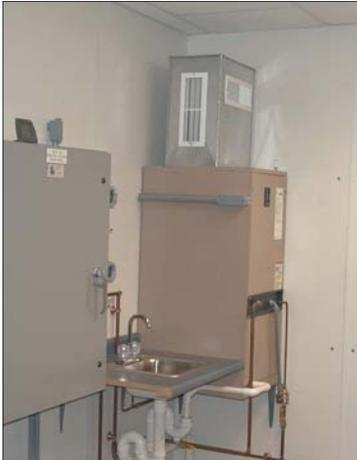
**The District saves thousands of dollars in power costs each year by using the naturally cool distribution system water to cool and dehumidify its booster and pump stations. A fully operational unit (corner mounted unit shown in above photo) typically runs under \$400 installed.**
