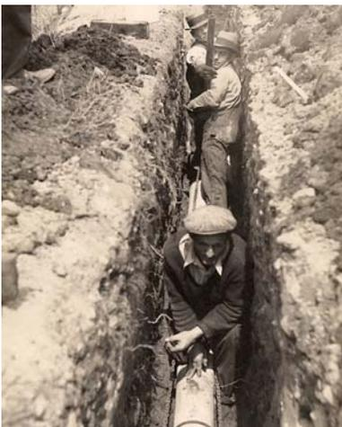
May 17, 1934 - District workers install the first Transite pipe used in Maine along Drakes Island Road in Wells. The 790-foot long project cost \$822.10, around \$1.04 per foot.
