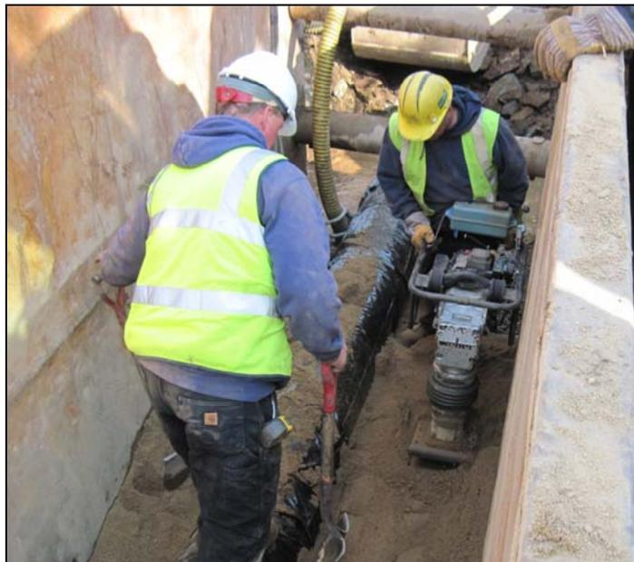
KKW Foreman Ed Thyng (l) and Josh Johnson (r) compact bedding sand around the new 16" ductile iron pipe on Skipper Joe's Point Road. The District wraps all ductile iron pipe with polyethylene prior to installation to guard against external corrosion.
