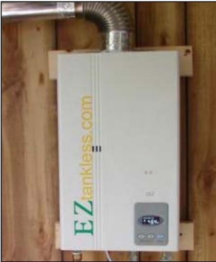
Tankless water heaters require minimal space and claim significant cost savings. However, owners are discovering they require regular maintenance to ensure proper operation. Many industry pros and manufacturers recommend these units be serviced annually by a qualified technician to remove calcium deposits that can decrease efficiency and restrict water flow. Calcium deposits can be flushed out of the water heater with vinegar.
