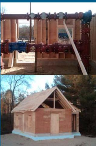
The new Arundel Booster Station on US Route 1 begins to take shape. Once complete, the new booster will enhance water pressure and fire protection along Route 1 in Arundel. All design and primary construction is being done "in-house" by District personnel.
