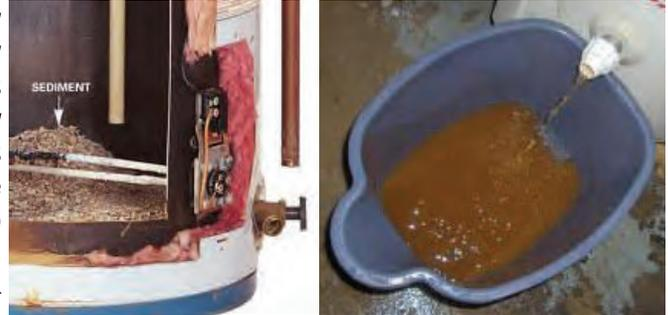
Hot water tanks are notorious for accumulating sediment and minerals, like iron and calcium (left photo), which can lead to aesthetic water quality issues such as color, staining, taste and odor. Hot water tanks should be flushed (right photo) every 1 to 2 years to help control the buildup of such deposits. The removal of deposits allows your water heater to operate more efficiently and extend its useful life. Contact your local plumber for assistance.
