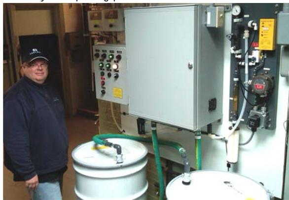
Bill Snyder stands next to the new chlorine dioxide system (ClO<sub>2</sub>) that was pilot tested for pre-disinfection of our Branch Brook surface water supply. The ClO<sub>2</sub>, which was installed by District staff, has worked so well to reduce disinfection by-products and improve aesthetic water quality that the District recently purchased the system for permanent use.
