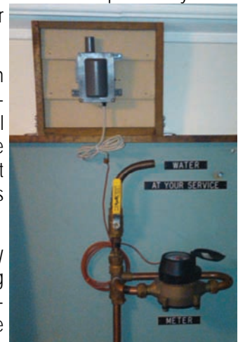
An example of a new AMR water meter (bottom) with exterior mounted radio transmitter (top).
