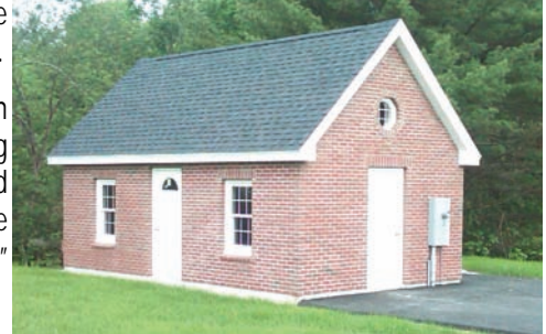
The new Arundel South Booster, designed and constructed by District personnel, is located on Route 1 at the Kennebunk and Arundel Town Line.
