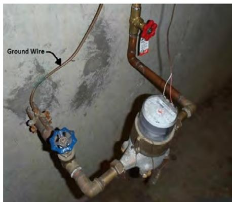
If your water service is being used for an electrical ground, there must also be one or two grounding rods installed outside.
