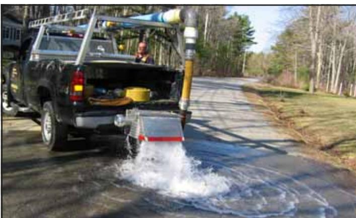
Assistant Utility Person Keith Archibald flows a hydrant at over 1,300 gpm to clean (scour) water mains and test fire flows during the "Spring Flushing Cycle." Mechanic Mark Lank built the custom diffuser which limits washouts and erosion while simultaneously recording flow rates and volumes.
