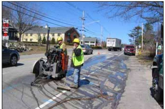
District crews saw cut 9" of pavement and 9" of concrete along busy Route 1 in Ogunquit prior to installing 1,680' of new 20" ductile iron water main. An additional 1,350' of new 20" main is slated for 2008 as a means to improve fire protection and system hydraulic capacity.
