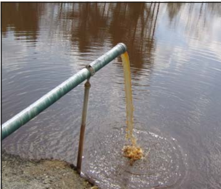
Step 1. Sediment is pumped from the District's treatment plant into one of its four "sludge" holding lagoons.
